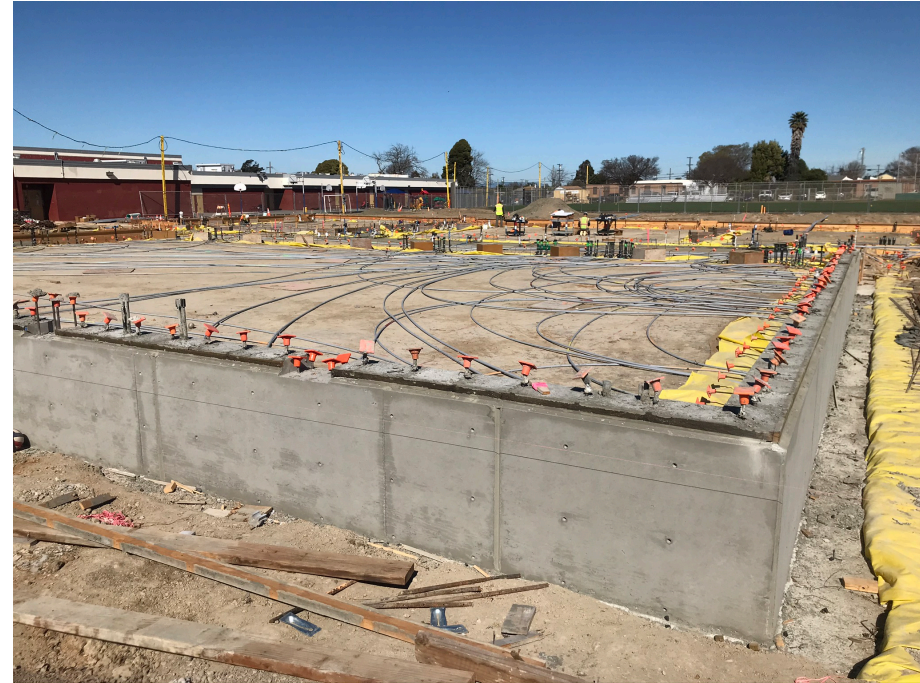
Gym Footing Stemwall
