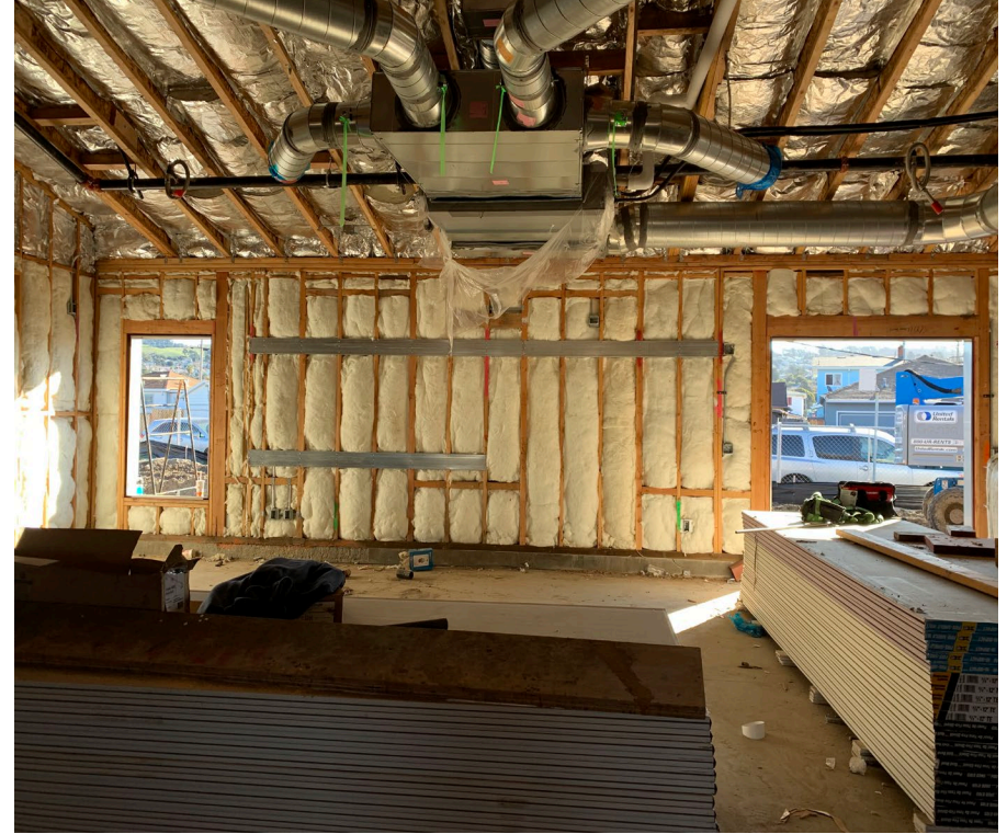
Library Insulation & Plaster
