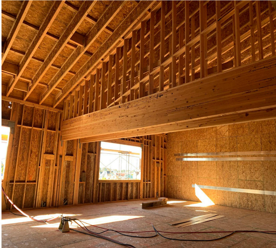
Learning Suite South Interior Framing
