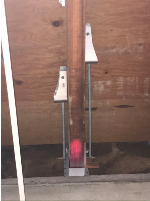
Seismic Braces, Science Bldg.
