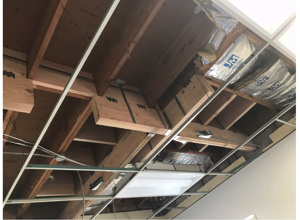
Seismic Blocking, Science Bldg.
