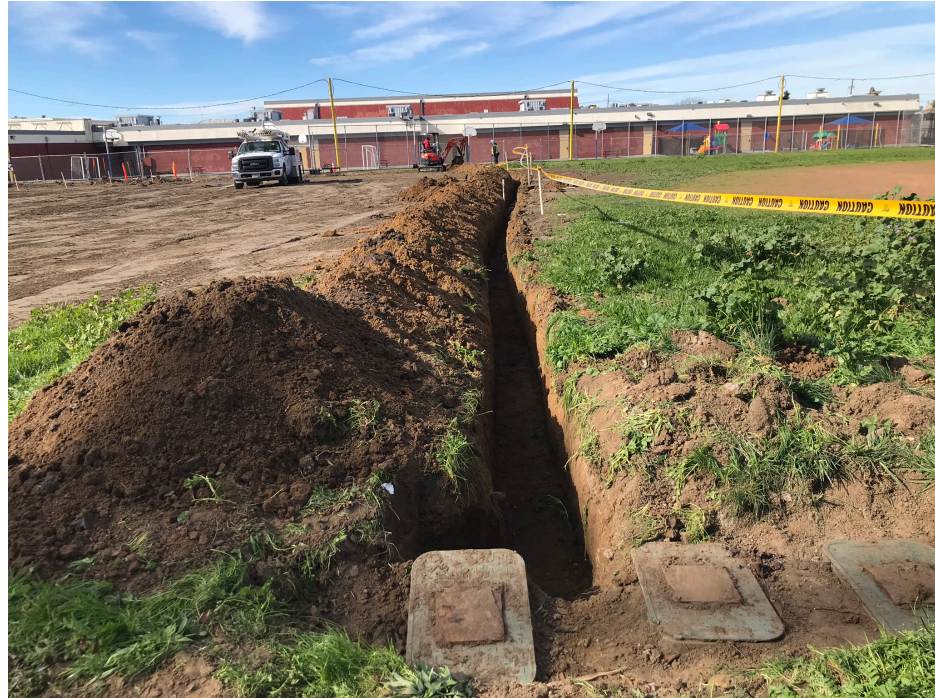
Softball Field Irrigation
