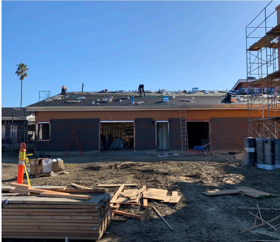
Admin Roof Shingle and Wall Lath
