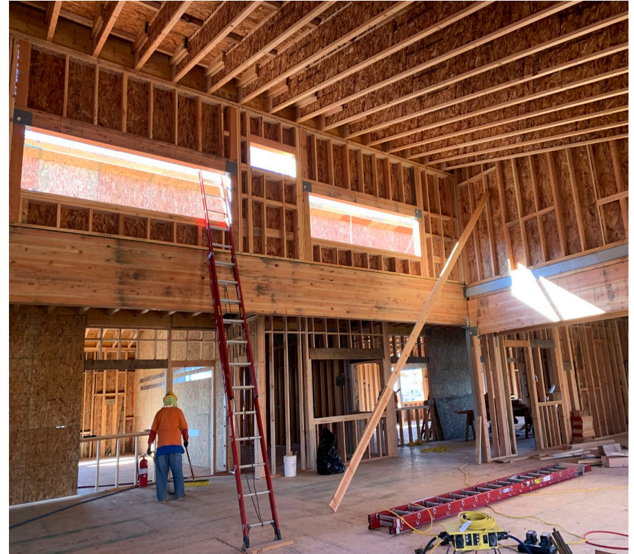
Learning Suite South 2 nd Floor Framing
