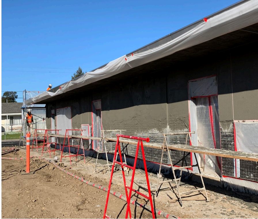
Kinder North Building Plaster
