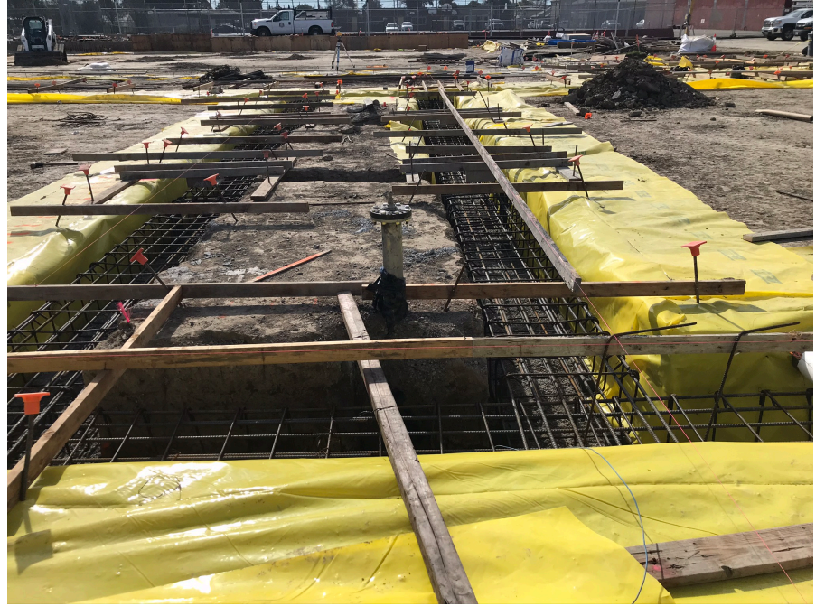
Gym Footing Rebar
