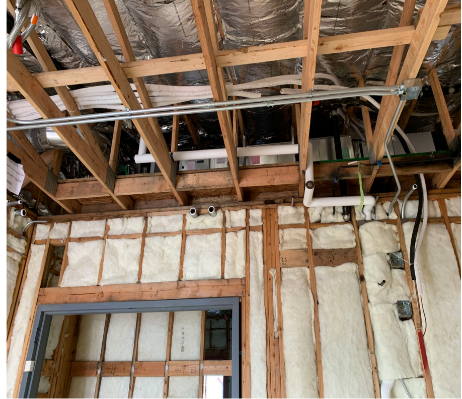
Kinder Room 111 HVAC Rough-In Above Ceiling
