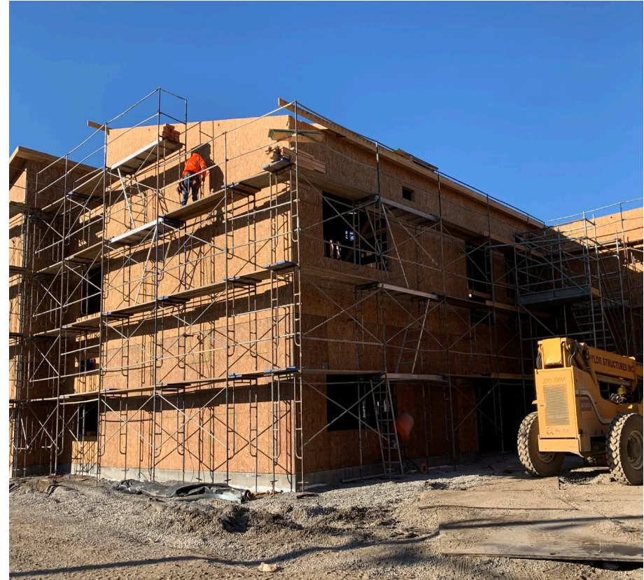
Learning Suite South Exterior Framing
